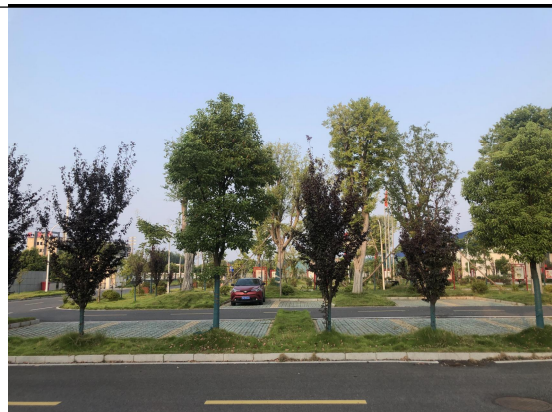
堆场区透水砖铺设
